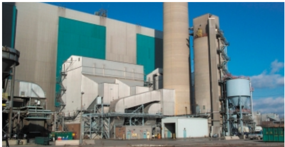
Figure 15 Electrostatic precipitators remove particles from the gases in large industrial facilities such as the one shown here.
